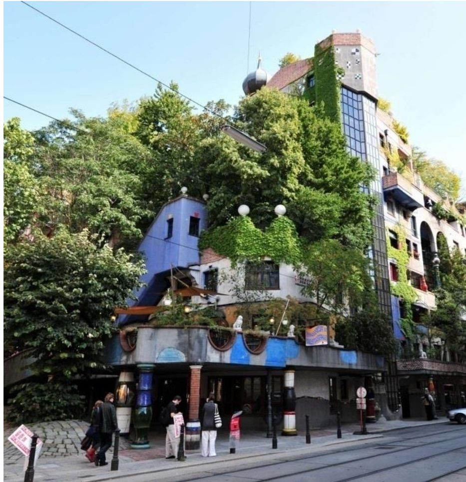
Pionier for greening buildings: Hundertwasser
